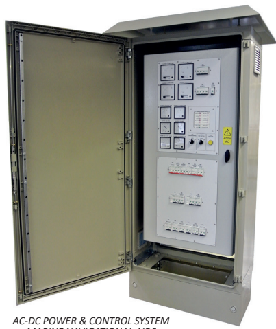
AC-DC POWER & CONTROL SYSTEM MARINE NAVIGATIONAL AIDS
